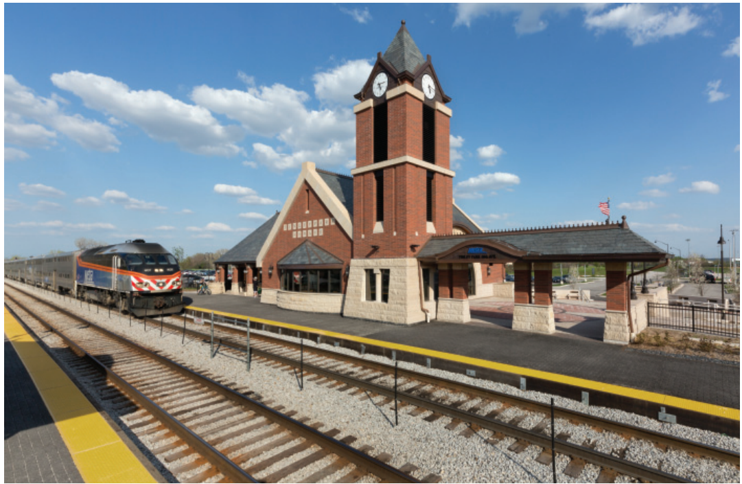
Masonry proportions, detailing, and decoration reflect traditional construction methods and create a sense of solidity and monumentality.
